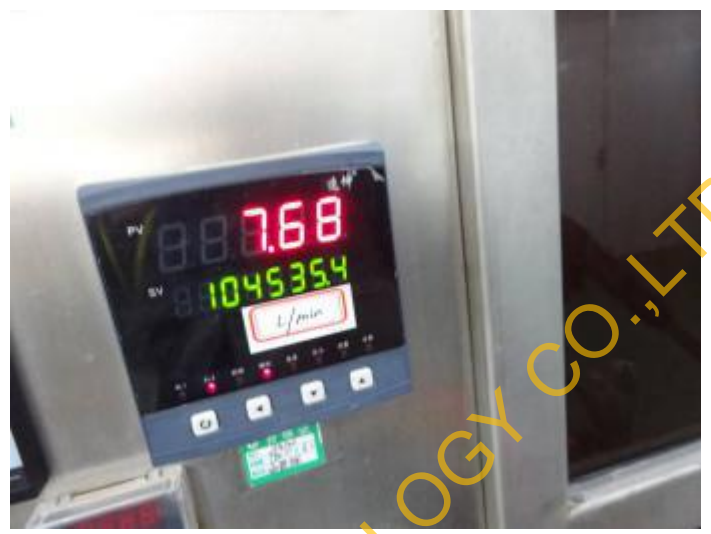
139. Max water Flow Rate Test
